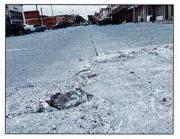
Chunks of street surface remain broken and missing, following structural failure of the resurfacing provided by Andale. The \$600,000 project was completed last year. (Photo by JT Strasn
