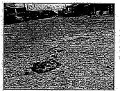
Chanks of street surface remain broken and missing, following structural failure of the resurfacing provided by Andale. The \$600,000 project was completed last year: (Photo by JT Strasner)
